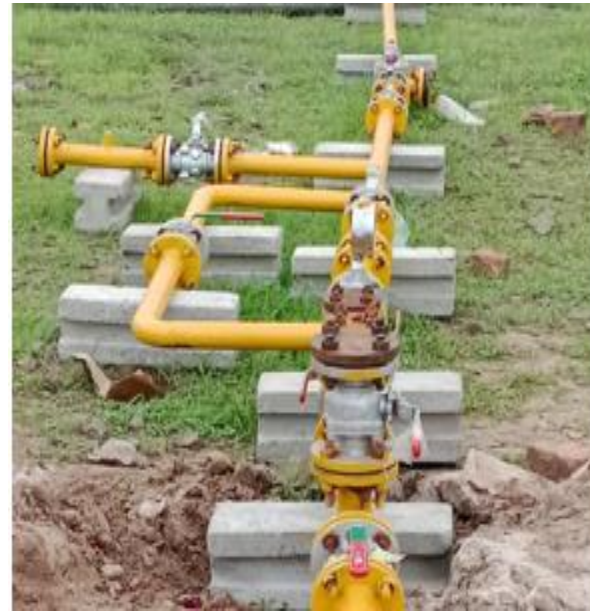
Gas Pipelines hookup to existing facility
