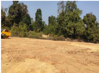
Site Grading and Fencing
