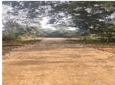
Approach road to wellsite
